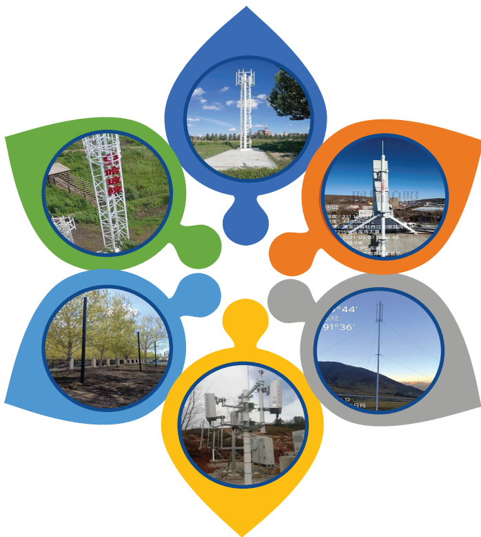
Telecommunications | Cellular Tower
