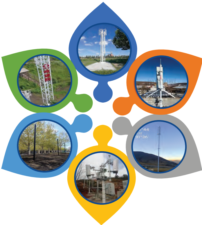
Telecommunications | Cellular Tower
